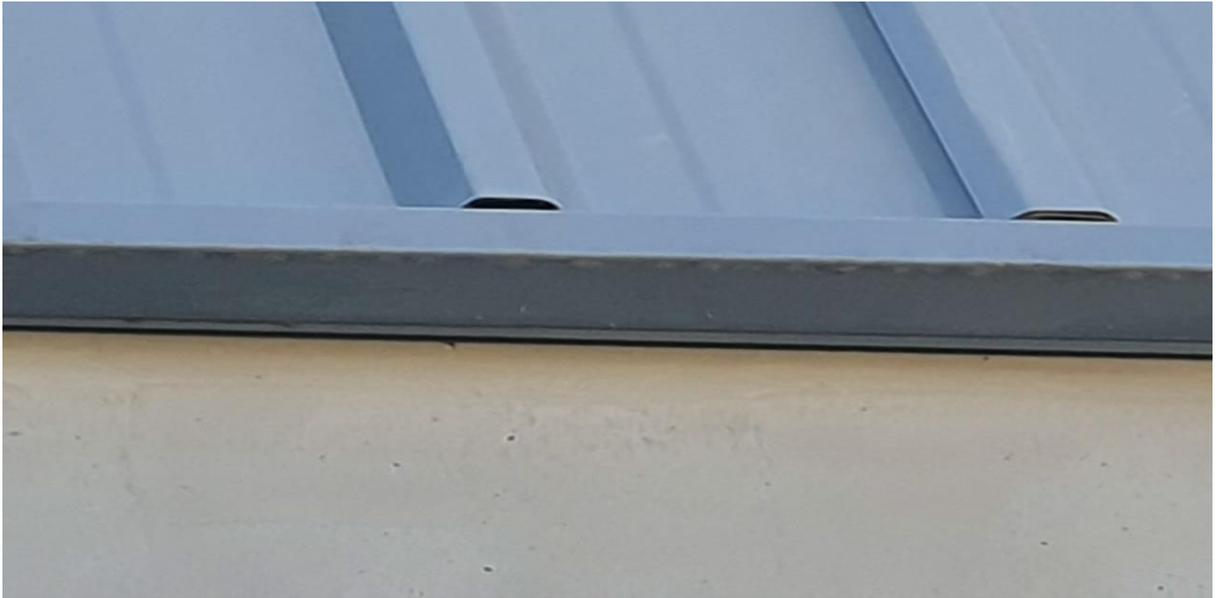
**Unpainted Alloy Finish , the surface forms variants of the surface oxides resulting in an inconsistent appearance.**
